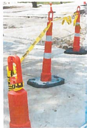
An elevated warning line, or barricade, in view of the operator must be erected.
