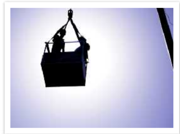
The operator-in-training cannot operate a crane if the crane is used to hoist personnel.
