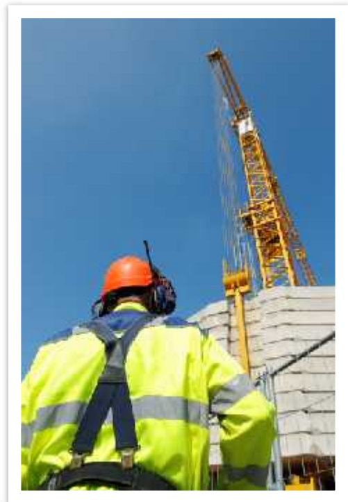
A crane operator often needs a signal person, to be able to operate safely.
