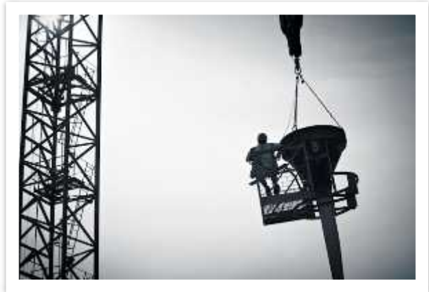
The personnel platform must be equipped with a guardrail system which meets OSHA criteria.
